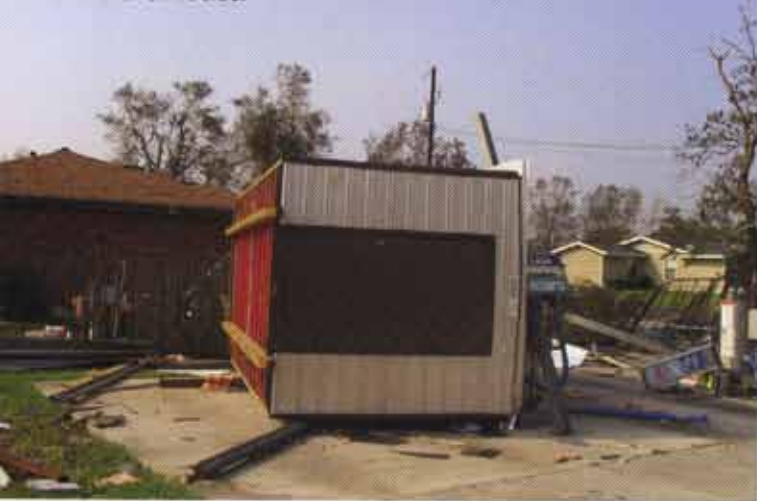
8x10 storage bldg. in West Orange blown over on its side.
